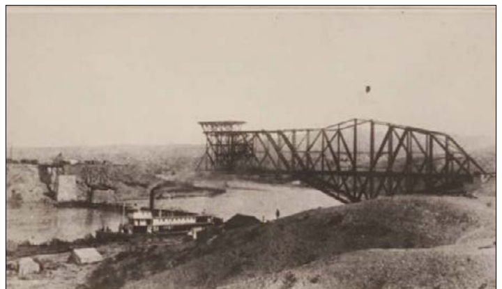
Building of the Topock Bridge, with the Gila steamboat. 1889 V103/126 The Otis Marston Colorado River Collection "The Huntington Library, San Marino, CA"
