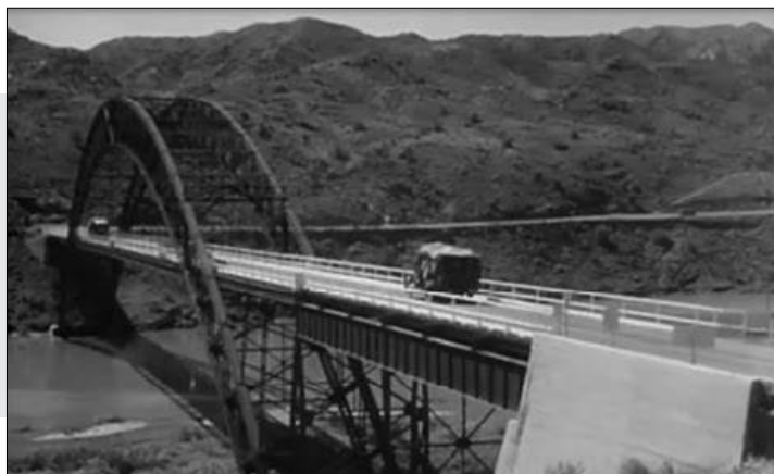
View of bridge and Route 66 from Topock. Notice how the road bed hugged the rocky area on the California side.
